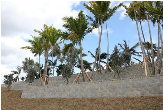
This site consisted of steep slopes below the interstate requiring multiple retaining walls in a terraced/tiered design on each side to create useable land for the planned landscaping. Allan Block's local representative reached out to Rob Cotleur, with [Cotleur & Hearing](#), on behalf of [PaverScape Inc.](#) to create a design for the retaining walls using Allan Block's new product AB Aztec Classic of the AB Aztec Collection.
