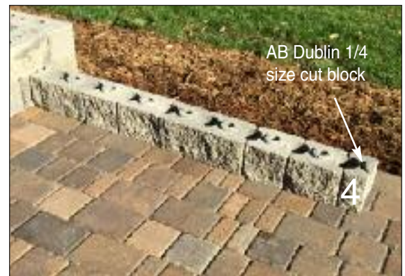
Ending at Corner
