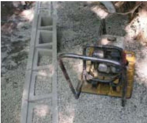
compacting the soil in "lifts" or layers. Compacting in lifts of 8 in. (200 mm) or less with the proper equipment and moisture content, will provide the necessary compaction. Compaction in lifts that exceed 8 in. (200 mm) will result in less than adequate soil strength. **Always backfill and compact after each course of 8 in. (200 mm) Allan Block is placed (figure 2).**
