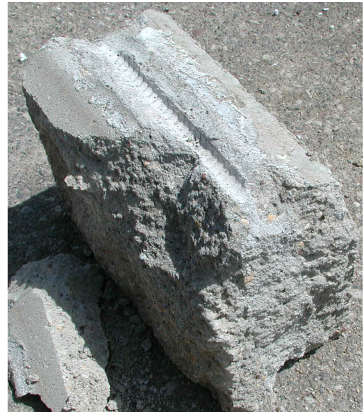
Figure 1: Sand Mix Grout in Panel Block
