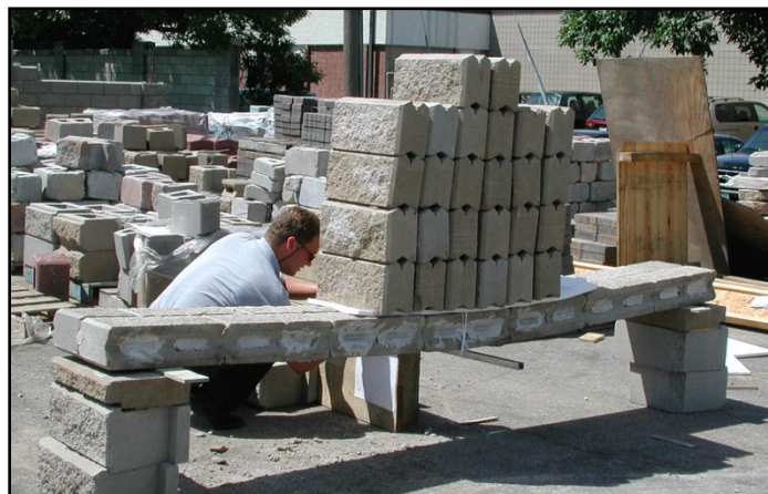
Figure 2: Loaded 7 Panel Bond Beam
