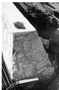
Mortared Stone Gravity Wall Malaysia
